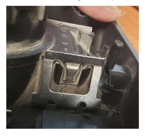
When installing the receptacles, make sure the DRVM unit opens DOWN. Pry the silver tabs out for a tight fit.
